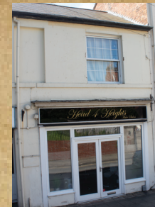
Location 9 - 10 Gloucester Street
