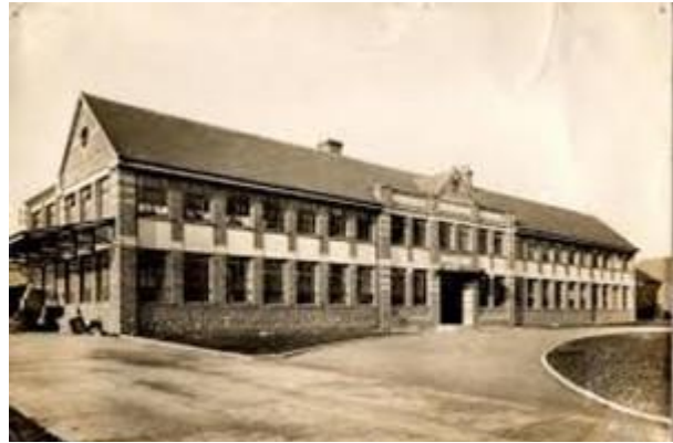
Tachbrook Road, Phase 1
